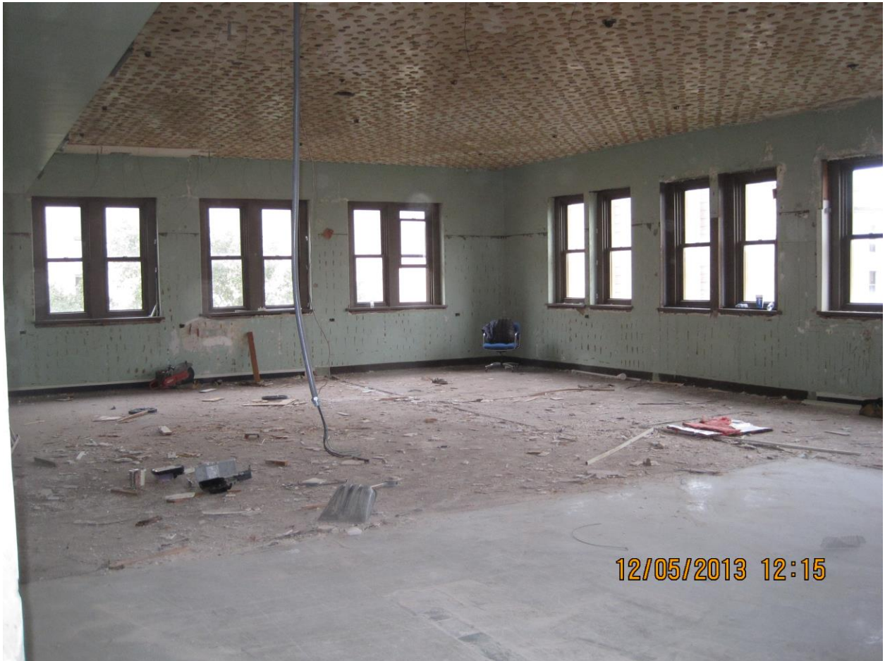
Third Floor Southwest Corner
