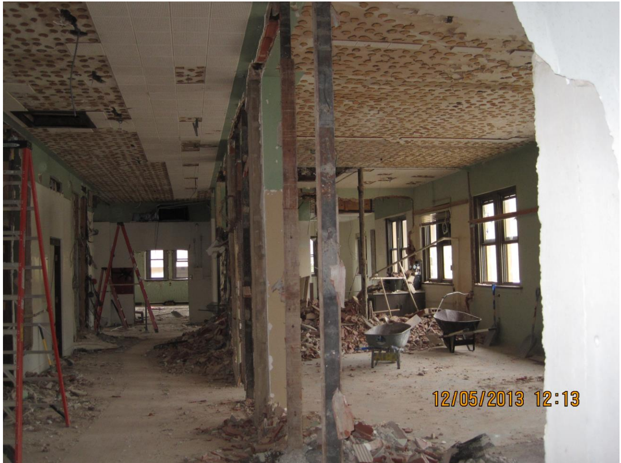
Third Floor Corridor
